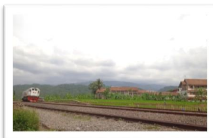
Figure 3. SMK of T2 is close to railway
